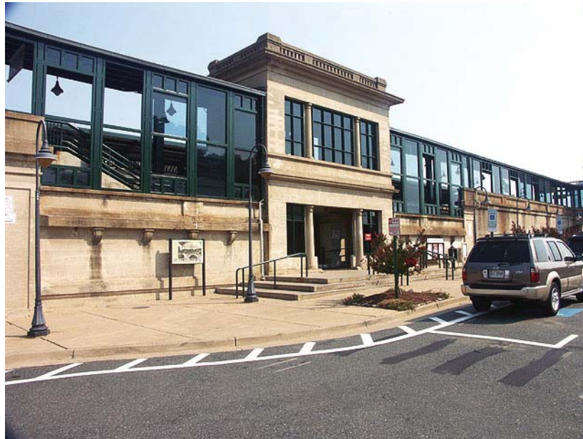
Plans are underway to rehabilitate the bridges surrounding the Fredericksburg Station.
