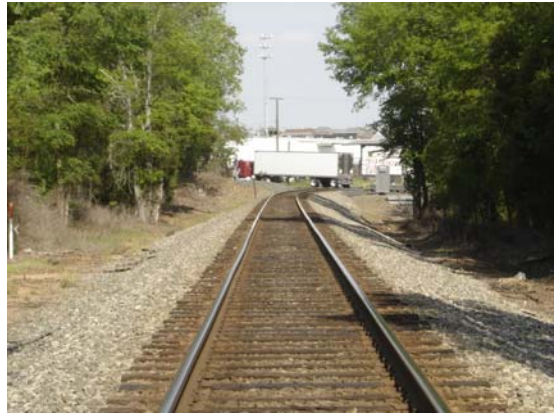
View of existing NS corridor.
