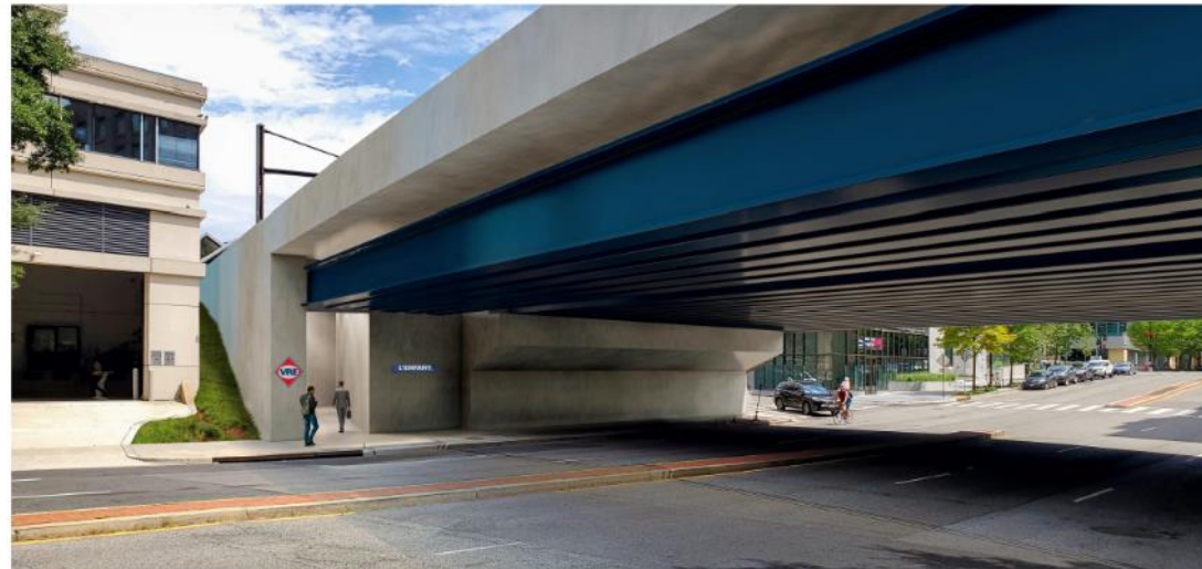
7TH ST SW TUNNEL ENTRY
