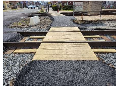
Temporary timber pedestrian crossing at the Quantico station.
