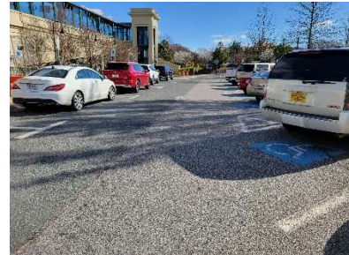
Fredericksburg station ADA parking lot (before upcoming improvements)
