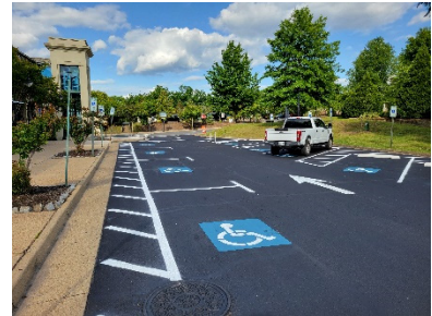
Sealcoating & restriping at Fredericksburg
