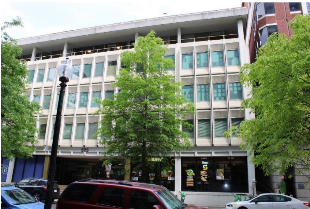
Photo 5. Partial view of the front (south) façade with recessed entrance on the first floor, facing north.
