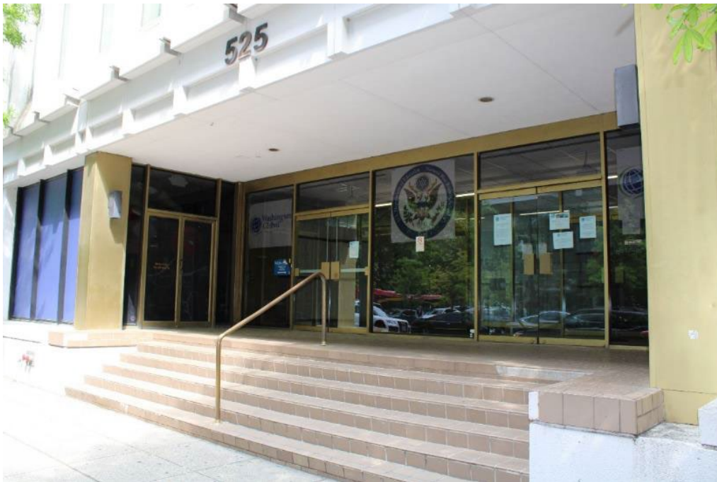
Photo 7. Detail view of the primary entrance, facing northwest.
