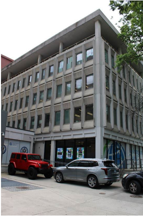
Photo 2. Northwest oblique view of the American Road Builders Association Building, facing southeast.
