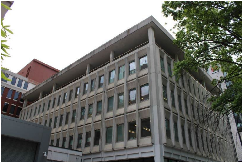
Photo 3. View of the upper levels of the north and west elevations, partially obscured by adjacent buildings, facing southeast.
