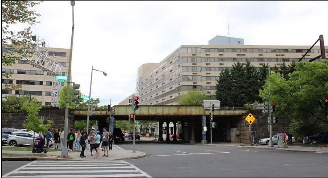
Photo 15. View of the south side of the 6 th Street Bridge as it crosses over 6 th Street SW at its intersection with Virginia Avenue SW, facing north (VHB 2024).
