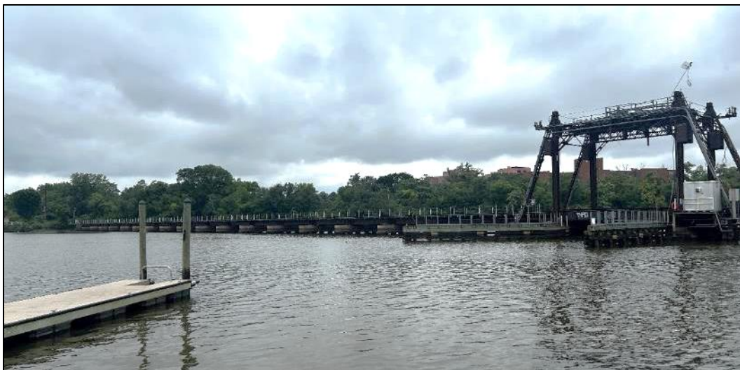
Photo 8: The Anacostia River Railroad Bridge as viewed from Anacostia Park, facing northwest (VHB 2024).
