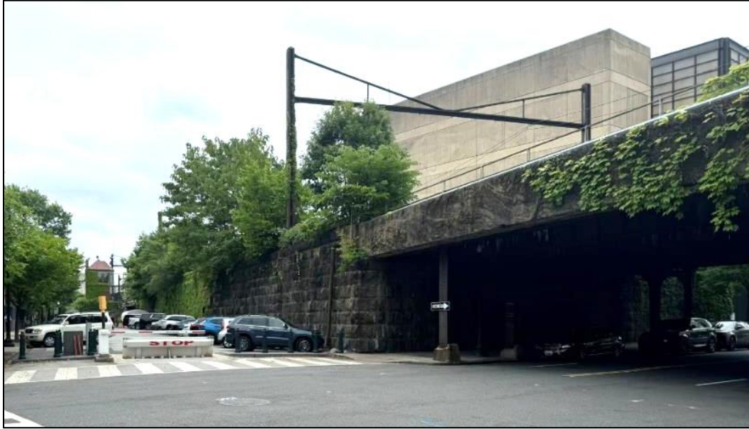
Photo 13: The 3 rd Street Bridge crossed by a pair of catenary poles as viewed from the intersection with Virginia Avenue SW, facing southeast (VHB 2024).
