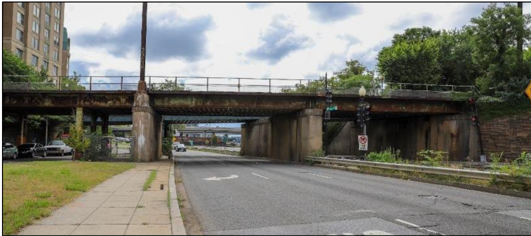
Photo 27. Maine Avenue SW Railroad Bridge, facing southeast (VHB 2022).
