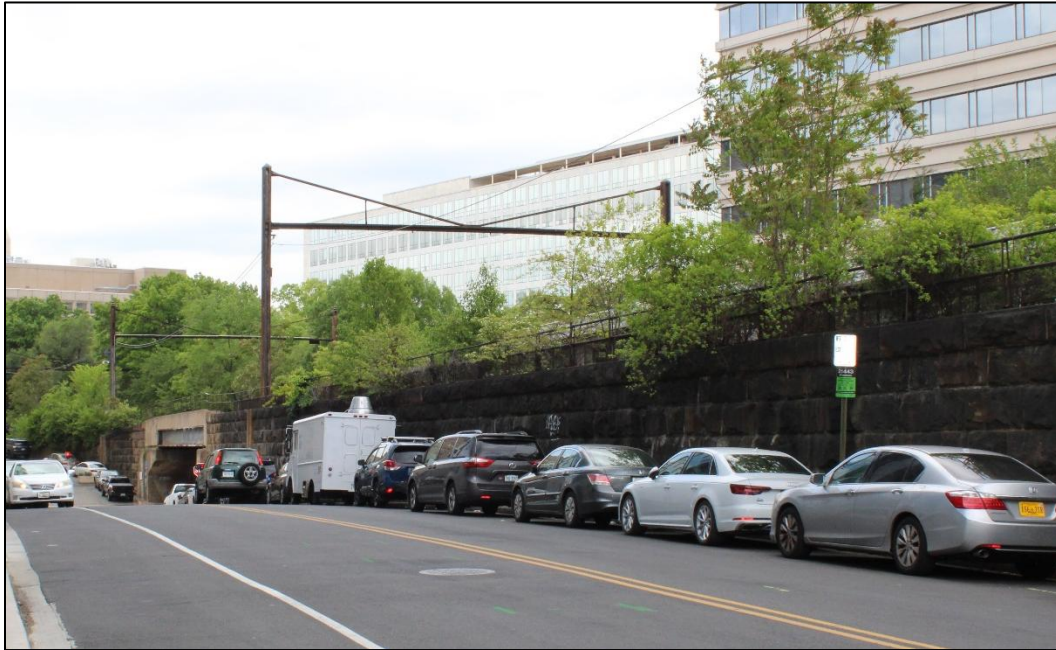
Photo 3: Catenary poles are visible crossing above the railroad tracks along Virginia Avenue SW near the 7 th Street SW Bridge, facing northwest (VHB 2024).
