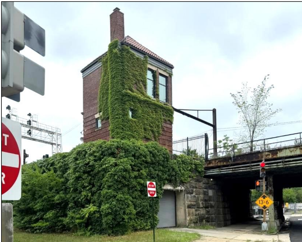
Photo 19: 2 nd Street SW Signal Tower as viewed from 2 nd Street SW, facing southeast (VHB 2024).
