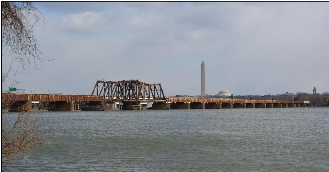
Photo 31: View of Long Bridge from the Mount Vernon Trail on the west shore of the Potomac River, facing north (VHB 2019).
