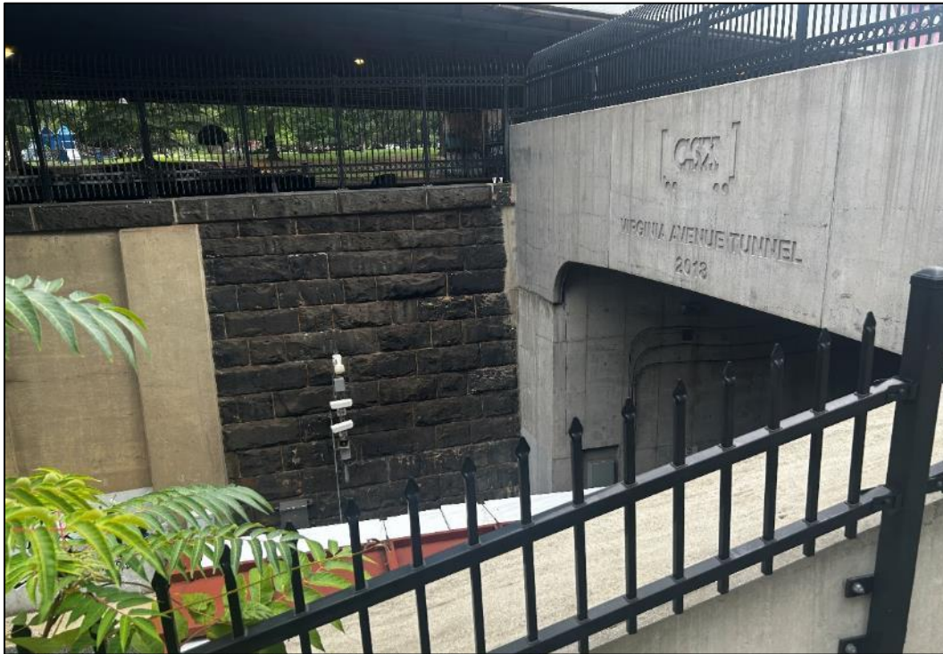
Photo 9: Western portal of the Virginia Avenue Railroad Tunnel as viewed from H Street SE, facing northeast (VHB 2024).
