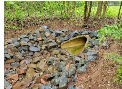
Drainage outfall rehabilitation at Crossroads MASF stormwater detention facility
