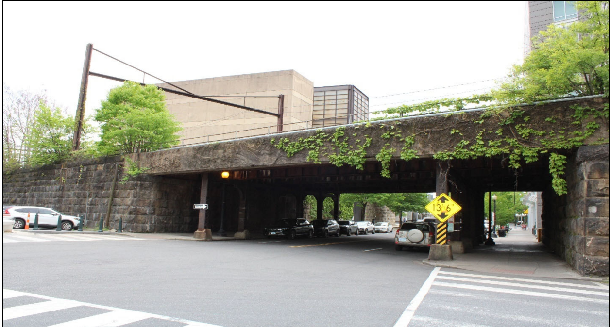
FIGURE 22. VIEW OF ELEVATED RAIL LINE ALONG VIRGINIA AVENUE SW, FROM 3 RD STREET SW, FACING SOUTH.
