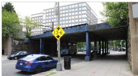
Photo 3-5: View of the c. 1903 6th Street SW Bridge looking southeast.
