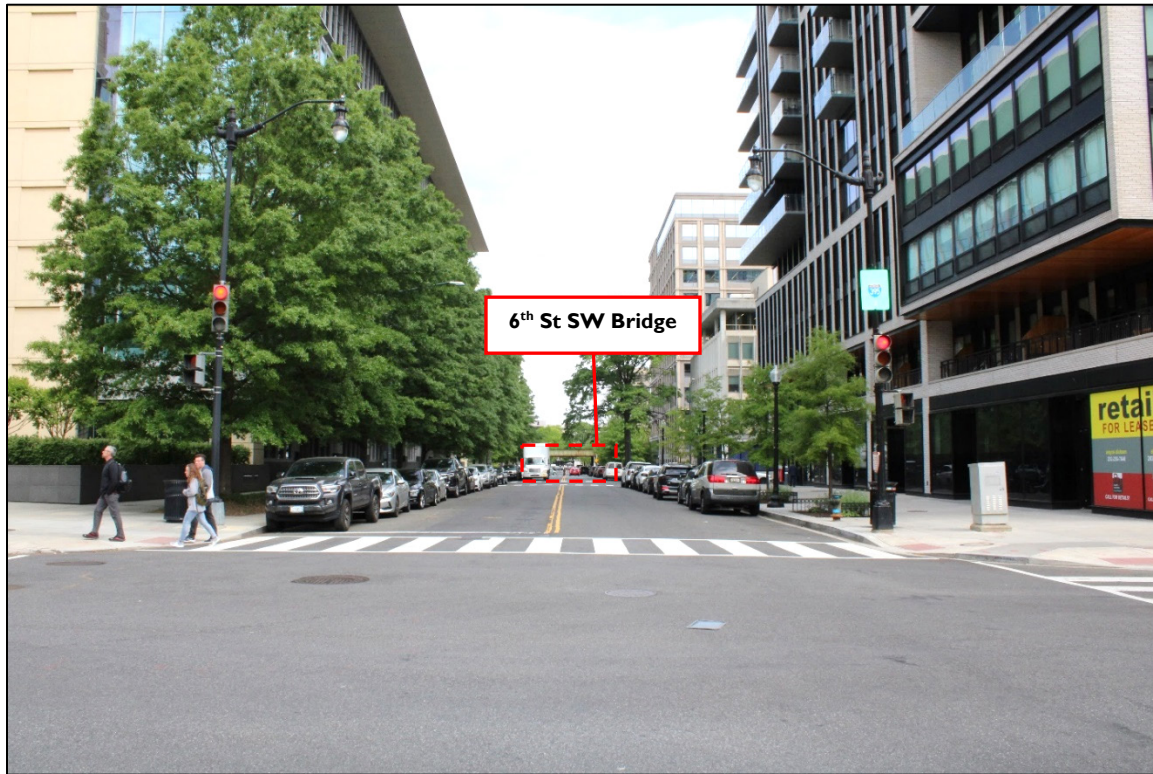
Photograph 11: View of the 6 th Street SW Bridge from the northeast corner of St. Dominic's Catholic Church. The bridge is visible but not a prominent part of the viewshed. Looking north along 6 th Street SW from the intersection with E Street SW.
