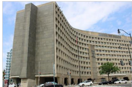
Photo 3-8: View of the southeast oblique of the HUD Building from intersection of 7 th Street SW and E Street SW.
