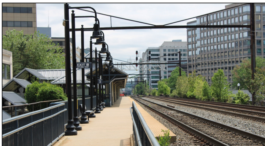
Figure 1-2: Existing Station Platform
