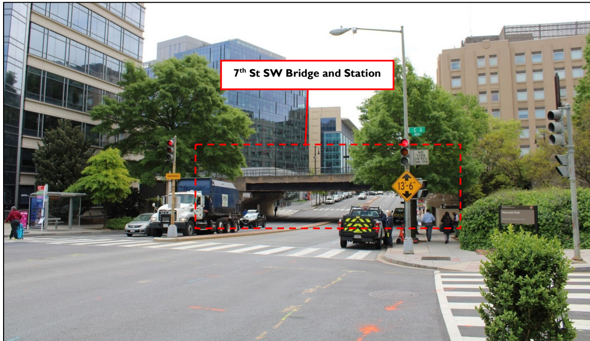
Photograph 5: View of the 7 th Street SW Bridge and L'Enfant Station from the southeast corner of the FOB 10A. The bridge and station elements are highly visible from this resource. Looking south along 7 th Street SW at the intersection of 7 th Street SW and C Street SW.
