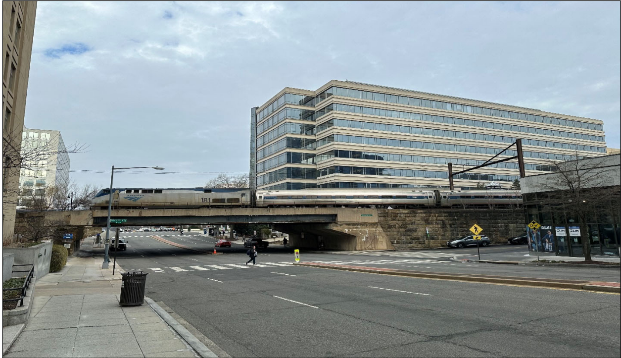
FIGURE 20. VIEW OF THE LOD FROM THE INTERSECTION OF 7 TH STREET SW AND VIRGINIA AVENUE SW, FACING NORTHEAST.
