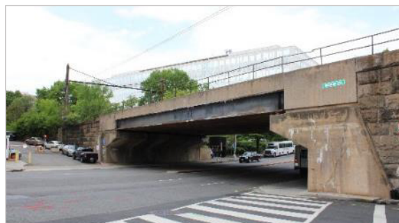
Photo 3-6: View of the c. 1970 7 th Street SW Bridge looking northwest.
