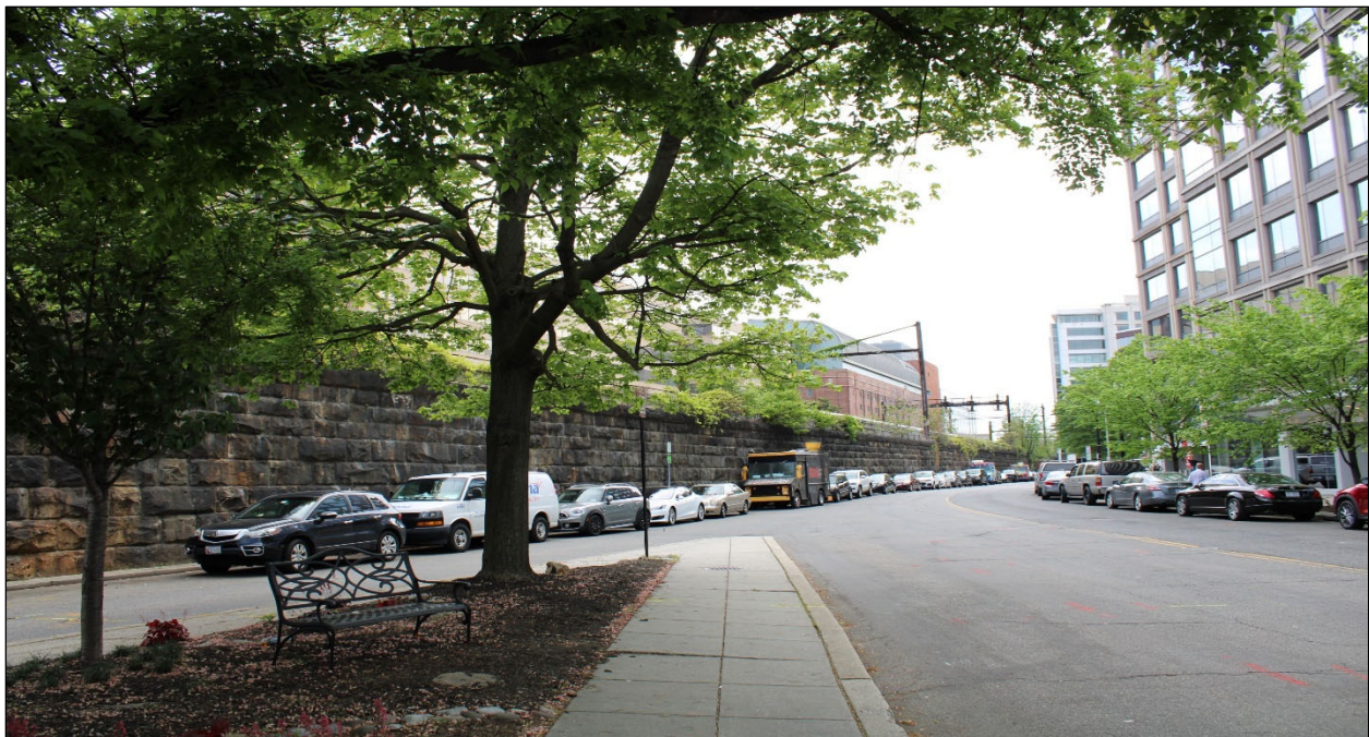
FIGURE 21. VIEW OF ELEVATED RAIL LINE ALONG VIRGINIA AVENUE SW, FROM 6 TH STREET SW, FACING WEST.
