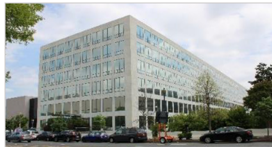
Photo 3-10: View of the southwest oblique of FOB 10B from 7 th Street SW.
