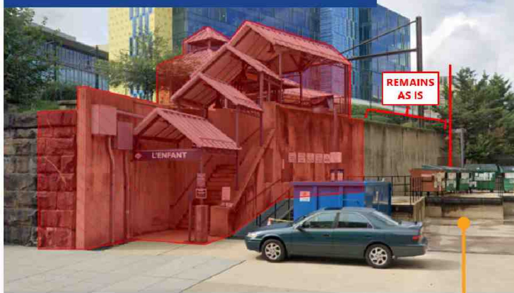
600 Maryland Ave loading area (Smithsonian office building)
