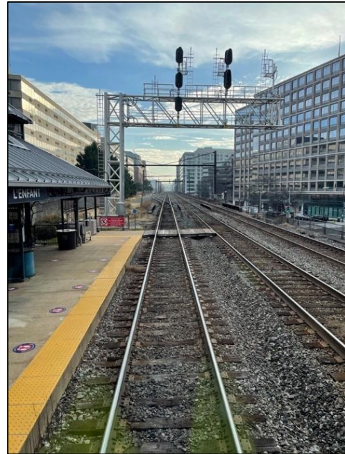
Figure 11- CSXT's Control Point Virginia Looking North Toward L'Enfant Storage Tracks
