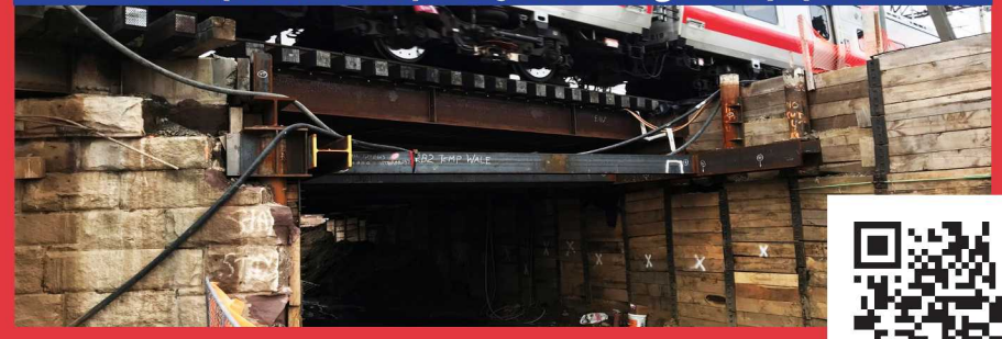
Example of a Temporary Rail Bridge Jumpspan.
